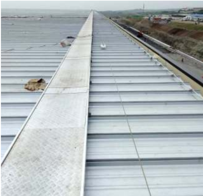
WALKWAY (CHEQUERED PLATE)
