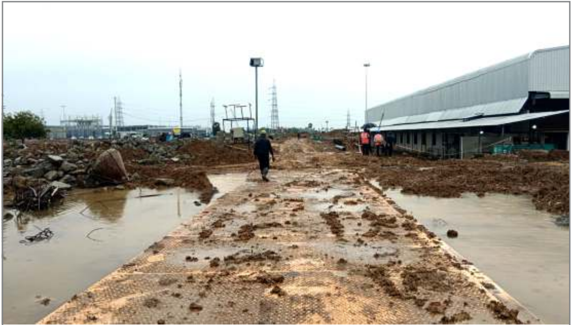
Area Each Mat: 4m x 2m Thickness: 94mm Material Strength: 425Ton/Sq.m Weight (Per Sheet): 360Kg.
