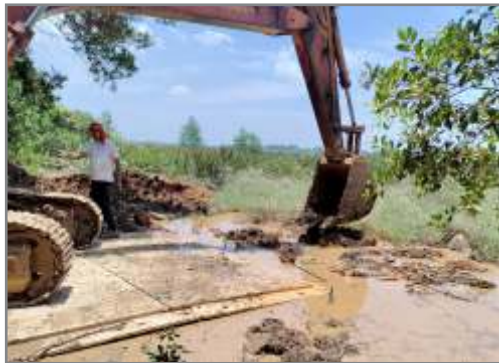
Area Each Mat: 4m x 2m Thickness: 94mm Material Strength: 425Ton/Sq.m Weight (Per Sheet): 360Kg.
