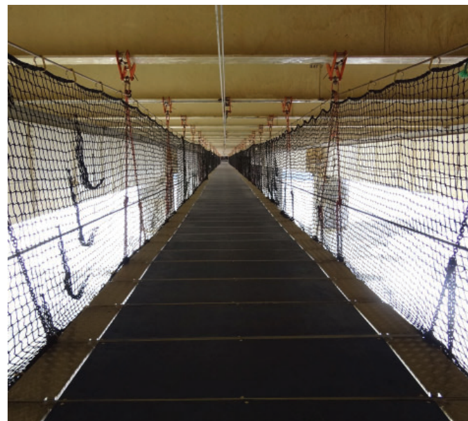
Complete bridge installation
