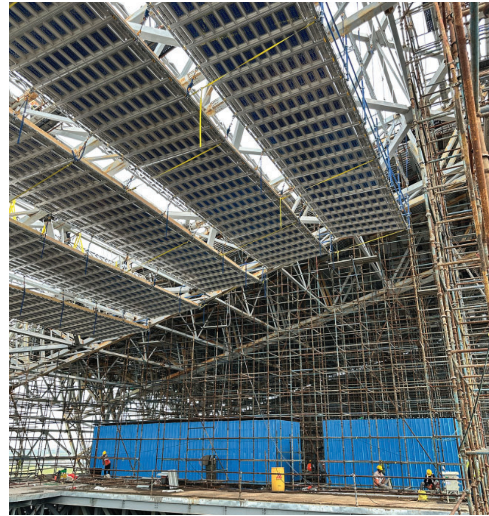
WEB Deck® stepped installation
