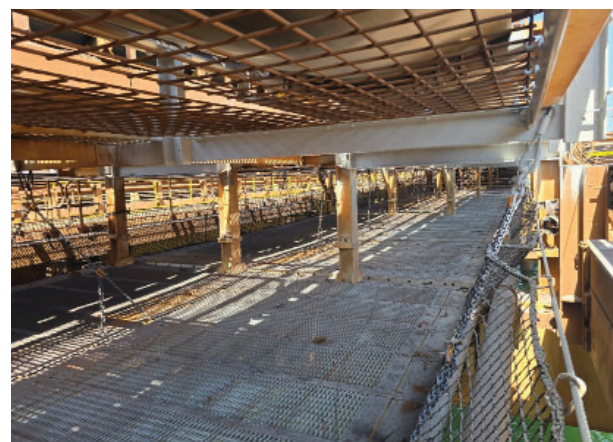
Grated deck installation
