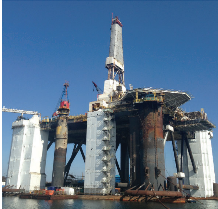
Full encapsulation of an offshore rig
