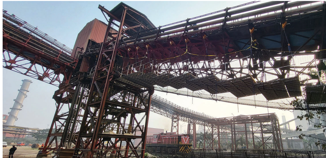
Stepped installation on a conveyor bridge
