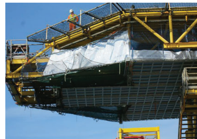
WEB Deck® offshore installation
