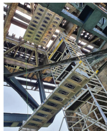
Ground up access
