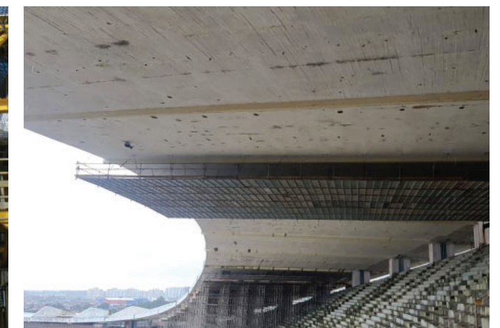
WEB Deck® arena installation
