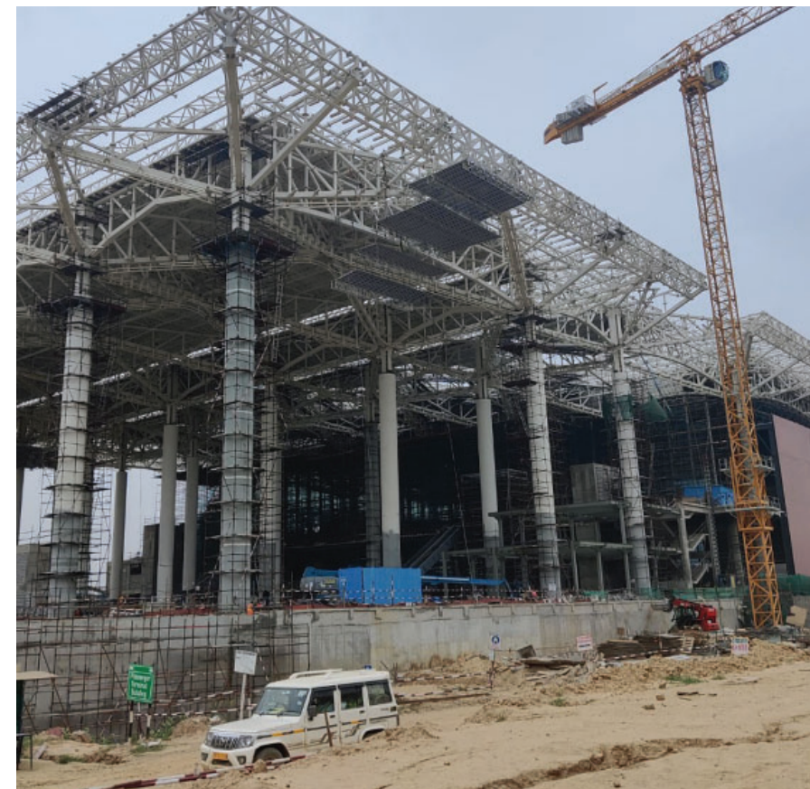
A stepped installation on a construction site
