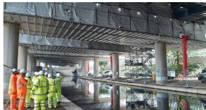
Bridge installation with WEB Deck®, WEB Net® and encapsulation
