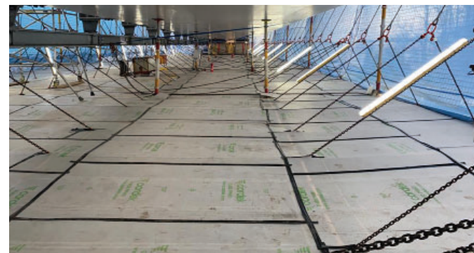
Complete bridge installation
