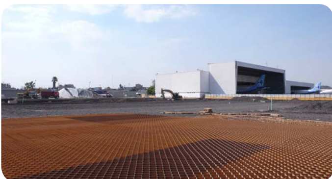
Large International Airport, Mexico Stabilized pavements over extremely soft soil
