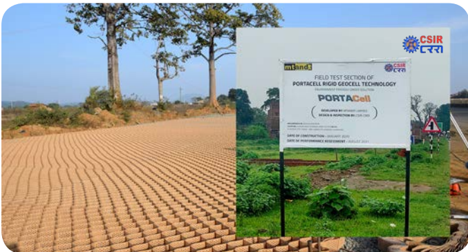
Khairatunda to Barwa Adda Section NH-02, Dhanbad Save upto 25% Asphalt thickness and 30% total pavement thickness
