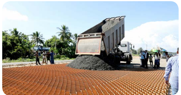
Vikravandi - Sethiyathopu (NH-45C) in State of Tamil Nadu Replaced unreliable chemically stabilized sub-base layer
