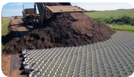
Paved and unpaved roads
