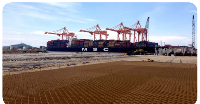
Load transfer platform stabilization in Ports, Latin America Use low quality infill to build durable pavements
